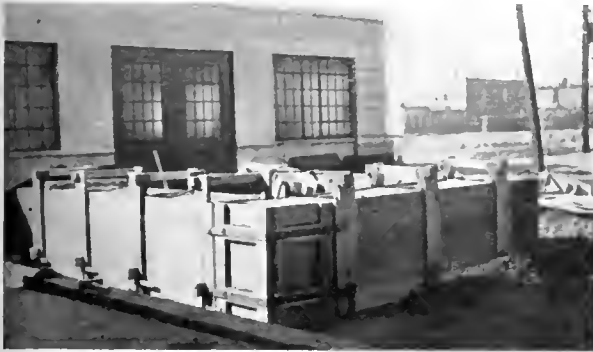
First Course—Shows form in place and filled with tamped earth EARTH HOUSE, ST. LOUIS, MO. THOMAS CRANE YOUNG, ARCHITECT
